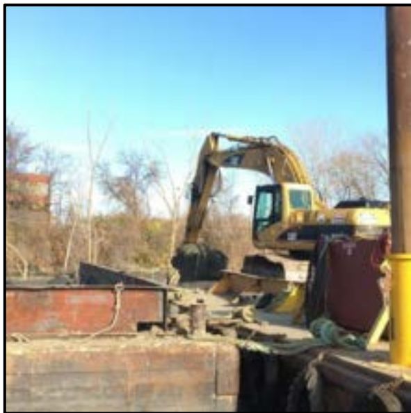
Figure 4: Mechanical dredging in the Maumee River.
