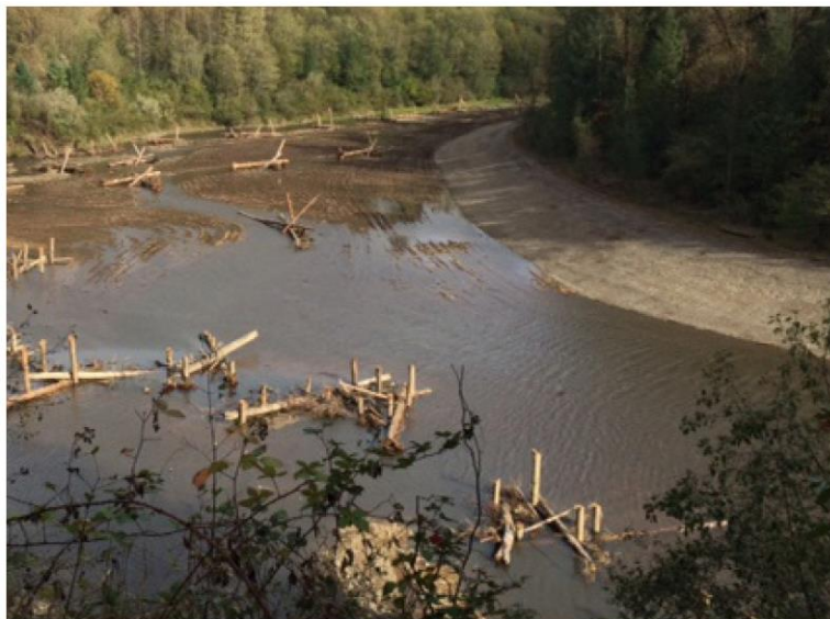
Figure 47: Woody habitat structure used in a large river system.
