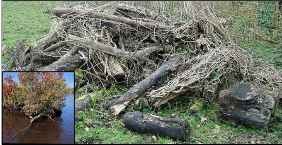
Figure 44: Logs used to contain dredged sediment. Logs would form the base of the planted hummock.
