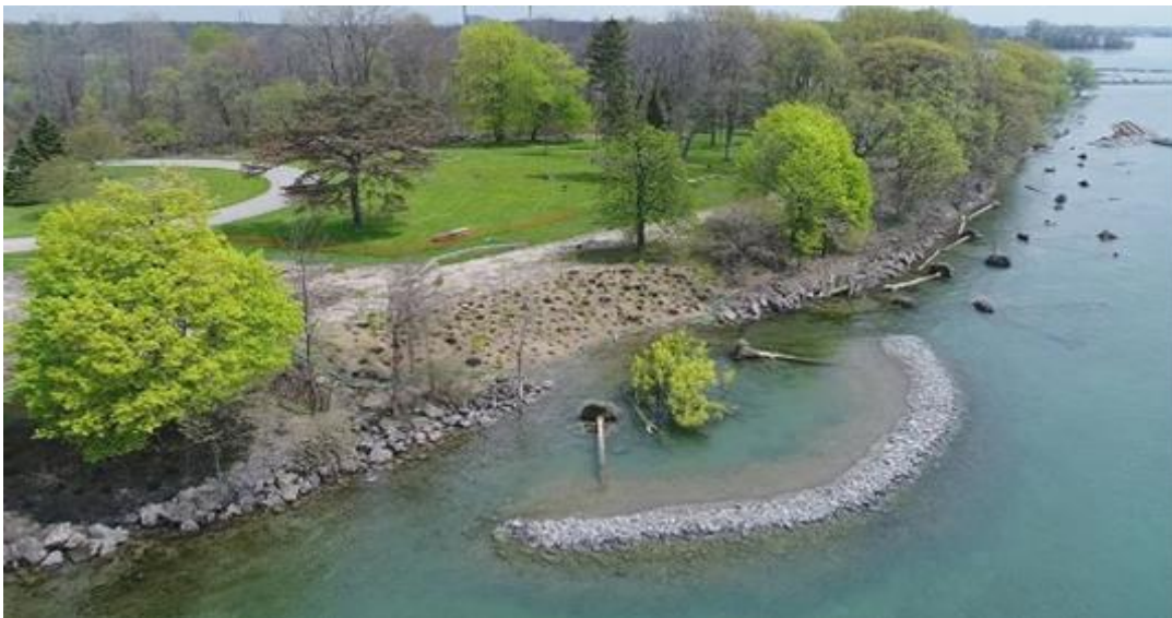
Figure 36: Rock reef and cabled logs/submerged trees. Source: Buffalo Niagara Riverkeeper.
